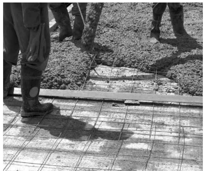
Pumping a concrete topping onto precast flooring. Reinforcement and screed battens in foreground.
