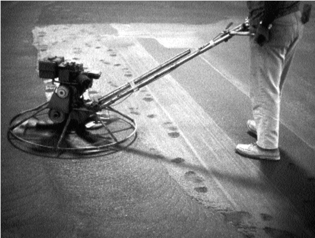
Power floating a screed.
